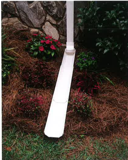
Downspouts should drain the water away from any impervious areas, such as the foundation or driveway, and into vegetated zones.
